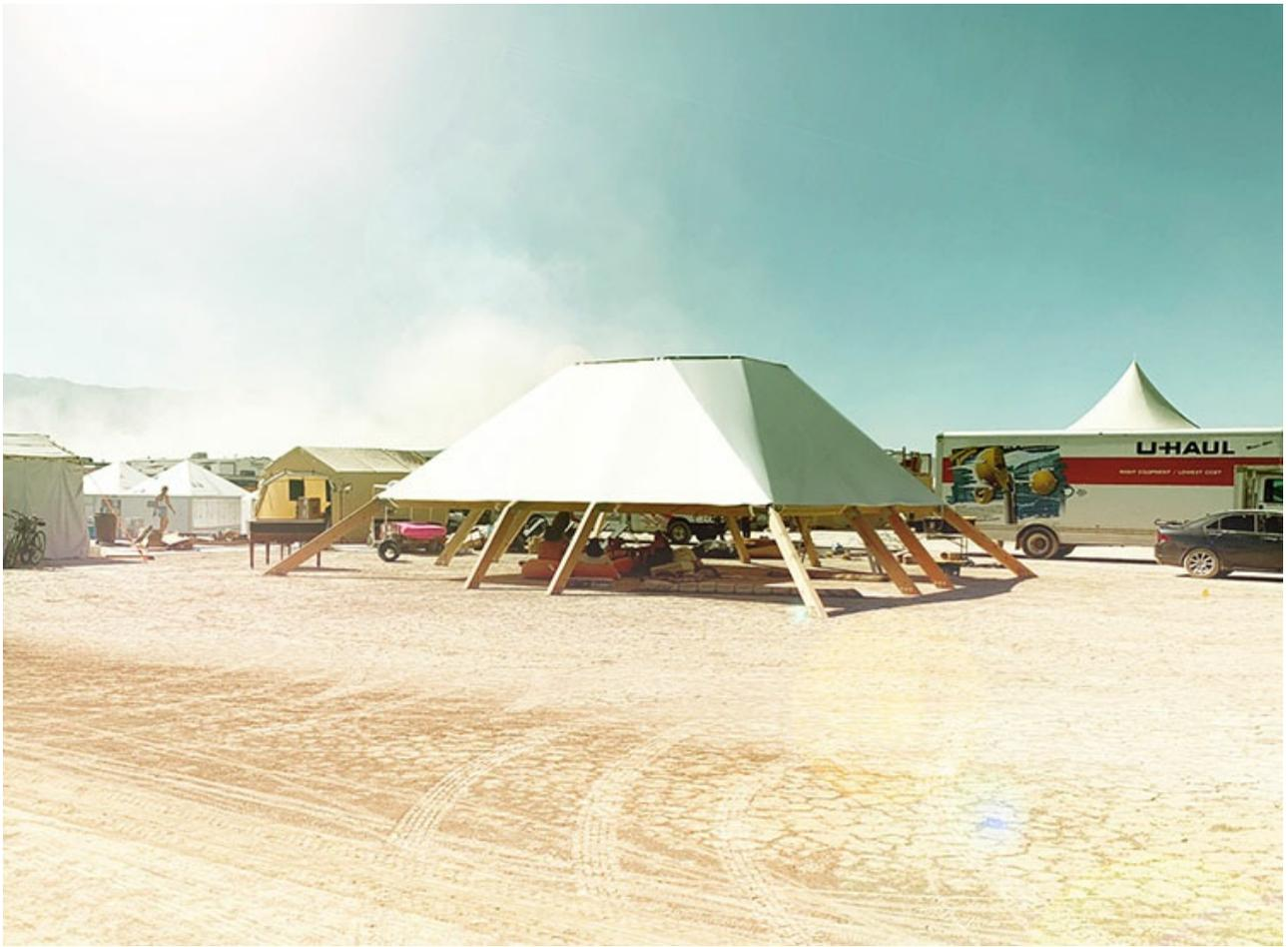
**By day the structure provides shade with an opening at the top that frames the Nevada desert skyline.** By night the opening provides ventilation for a central fire for *F Camp* members to gather around. The structure was designed to feel open from a distance and intimate when inside, achieved by elevating the structure off the ground.
